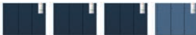
In conventional operating mode, the active A/C units run continuously at full load. The standby unit remains unused.
