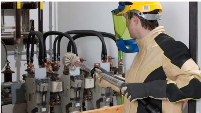
Live cleaning of a transformer using the TRS MS dry cleaning kit.
