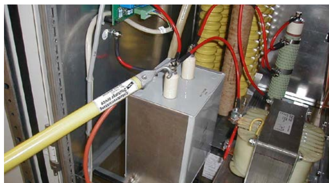
Single-pole device for discharging static charges
