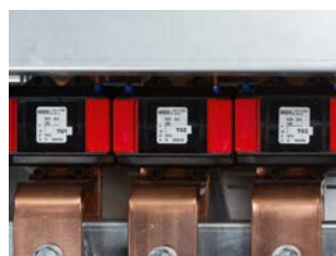
Built-in protective current transformers
