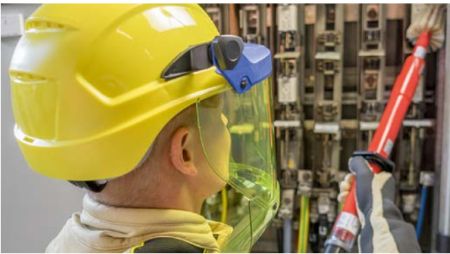
Electrician with necessary protective equipment.
