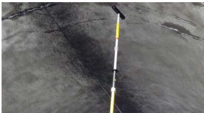
Removing icicles on a tunnel entrance.
