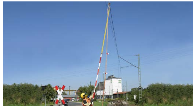
Attaching a railway earthing device.
