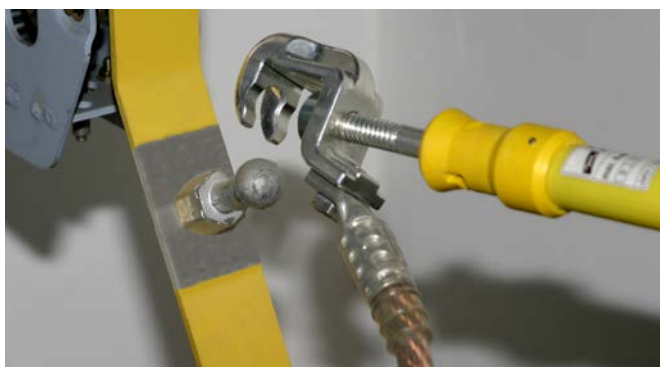
Connecting the phase cable end with universal clamp to a fixed ball point
