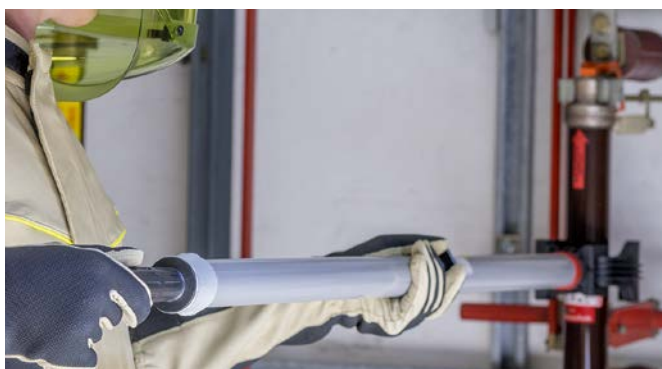
SZ fuse tongs for inserting and removing HH fuses
