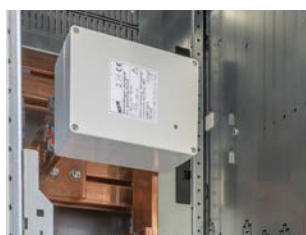
Built-in quenching devices
