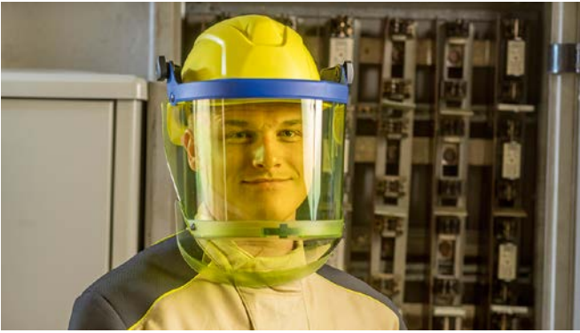
Installer in a low-voltage switchgear installation.
