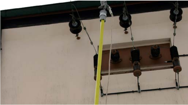
Telescopic earthing stick with aluminium cone coupling and phase screw clamp.
