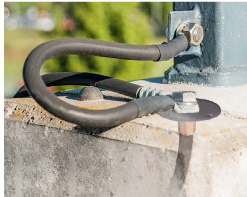
Fig. 3: Earthing connectors
